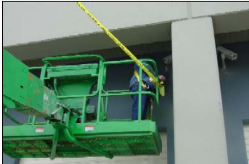
View of aerial platform during OR-OSHA investigation.
