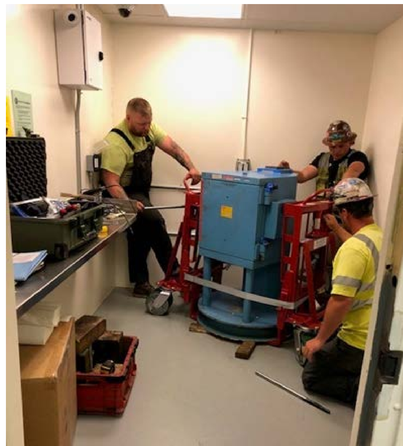
Cesium irradiator removal on Marquam Hill
