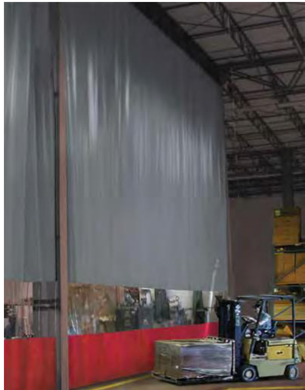
Image 7. Example of a retractable warehouse curtain wall, that would create a physical barrier between pallet rows, while also allowing for visibility through curtain wall at pedestrian or forklift operator height. Photo credit: TMI, LLC warehouse partitions sales brochure (TMI LLC, 2020).
