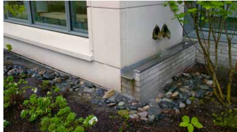
Water drains outside of BRB on OHSU Campus
