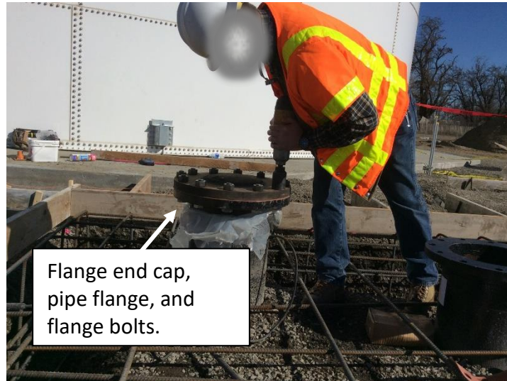
Photo 2. Simulation of work performed by victim prior to incident. Note backfill and rebar lattice. (Photo courtesy of OR-OSHA.)
