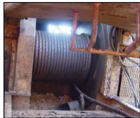
Additional torque on the line due to the far extension of the guylines and the reduced diameter of the drum may have helped topple the tower.
