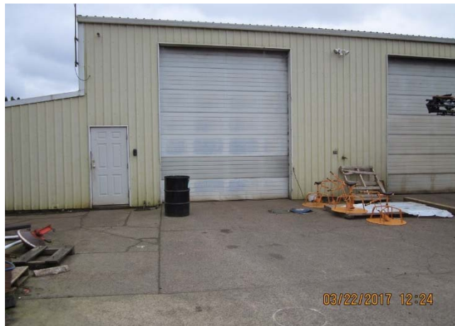
Photo 1. Shop exterior; bay door reportedly had been partway open at time of incident, presumably for ventilation ( Photo courtesy of OR-OSHA ).
