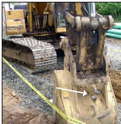
latched hook welded onto the quick-coupler to replace the original closed "lifting eye" supplied by the manufacturer.
