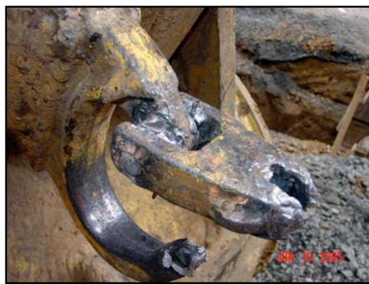
Part of the latch remained attached to the hook welded on the Hendrix Quick Coupler on the arm of the track-hoe.
