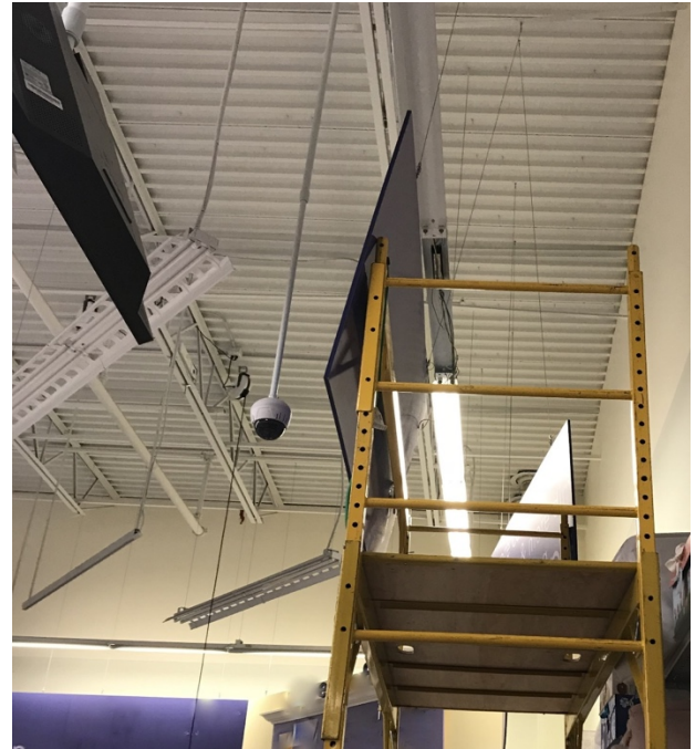
Image 7. Different angle of light fixtures and signage suspended from the roof by metal braided wire. Scaffold location recreates where decedent was working at the time of the incident.
