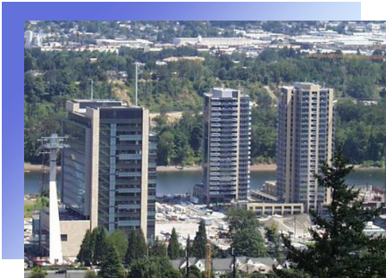
Left Bldg – OHSU Family Medicine at South Waterfront – 9 th Floor, Center for Health & Healing (CHH) Pennington Lectures – CHH 3 rd Floor
